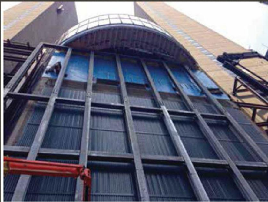
Figure 3. Vierendeel truss.
