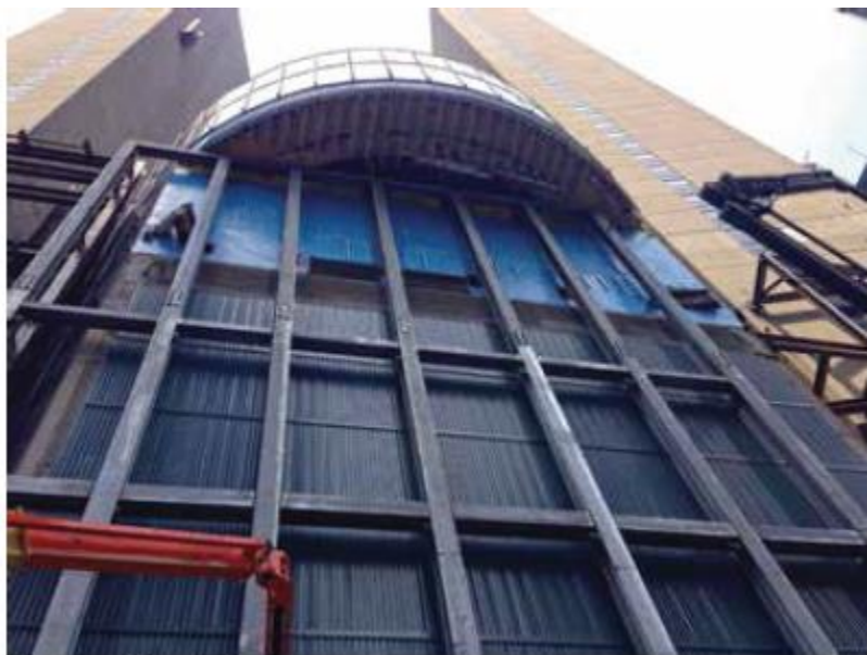
Figure 3. Vierendeel truss.
