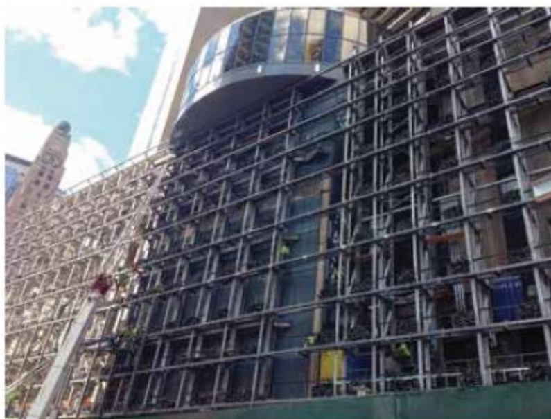
Figure 4. Installation of LED sign.
