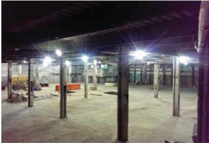
Figure 5. New double story space with reinforced columns.
