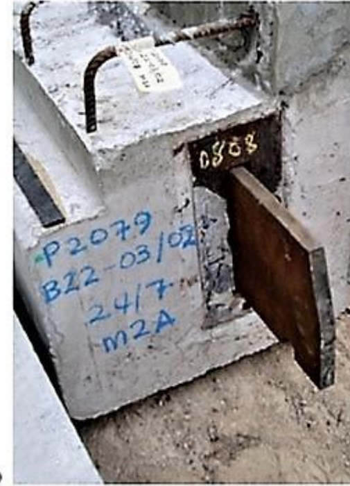
Figure 7.69 (a) Sliding plate connector steel plate is expressed from the beam after casting, and (b) is received into the steel box slots in the column.
