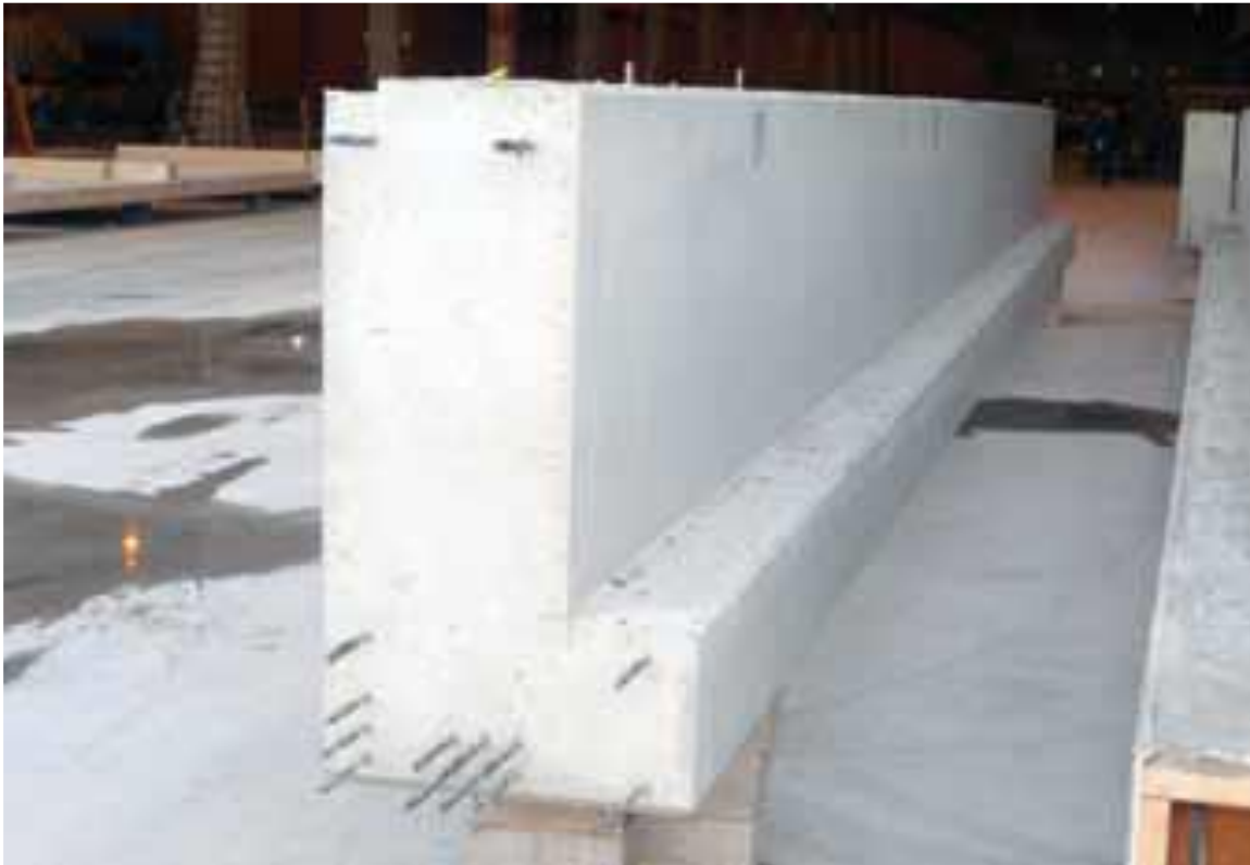
ledger beam(L shaped beam)
