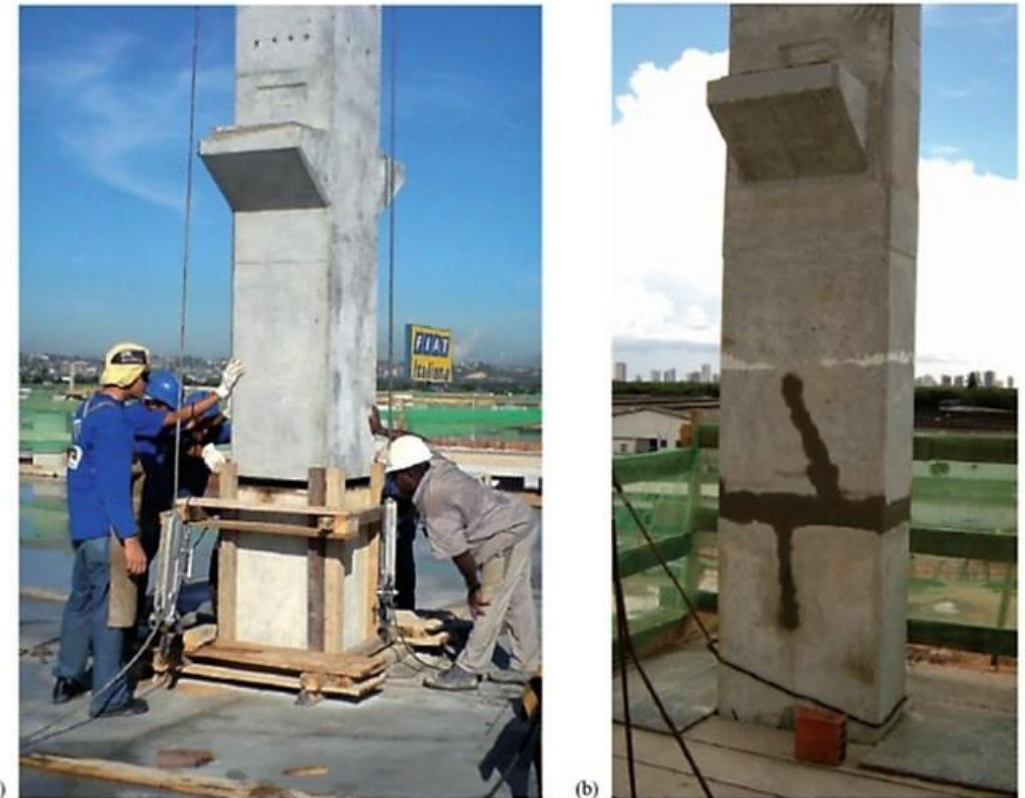
Figure 7.108 A welded plate column splice: (a) alignment using templates and yokes, and (b) completed joint. (Courtesy of T&A Prefabricados, Recife, Brazil.)
