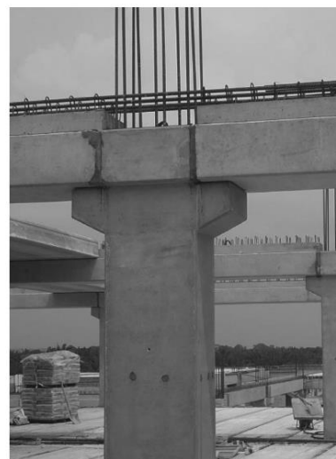
Figure 9.5 Precast concrete column corbel.
