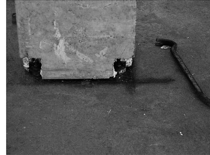
Column shoe in precast column construction.
