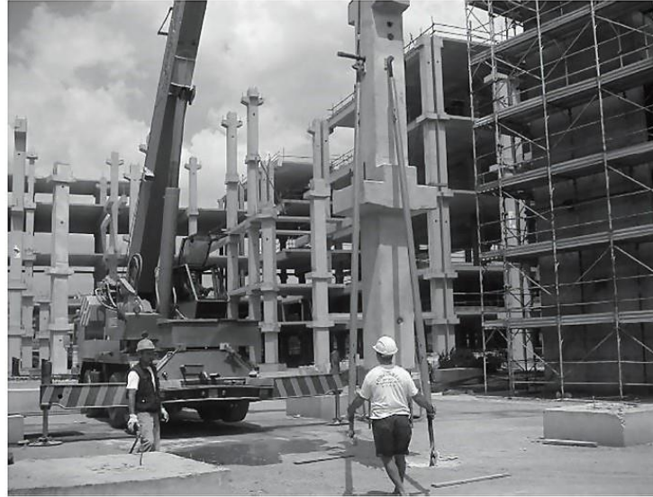
Pitching columns up to six storeys in height.
