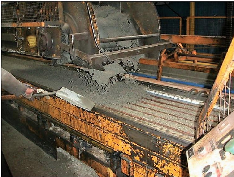
Figure 5.52 Second pass of the semi-dry concrete mix to manufacture reinforced hollow-core slabs. The top of the mould is the bottom of the slab. Manufactured by Creagh Concrete, N. Ireland.
