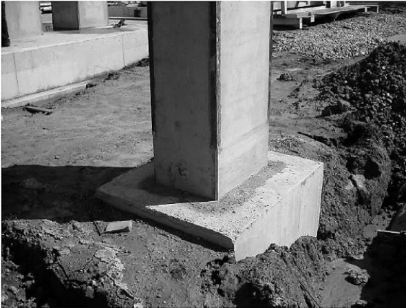
Column-to-foundation connection using a grouted pocket.
