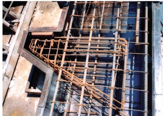
detailing in a shallow corbel.
