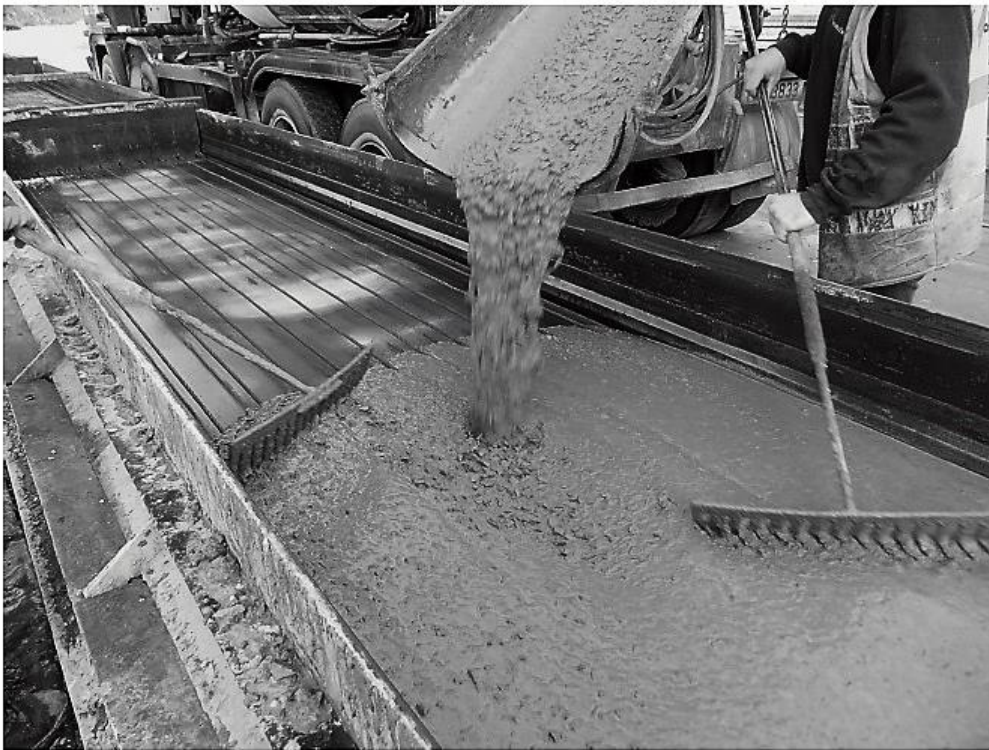
Self-compacting concrete, flowing and compacting without segregation, used to manufacture prestressed floor slabs.
