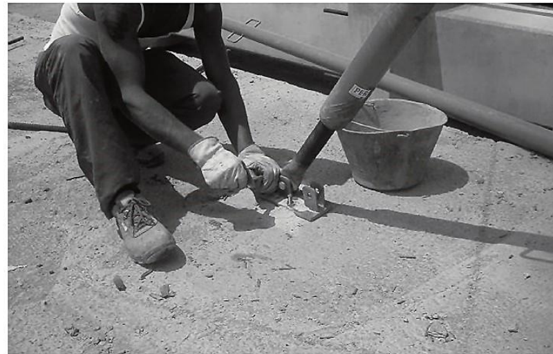
Securing the bottom of the prop to the ground beam.
