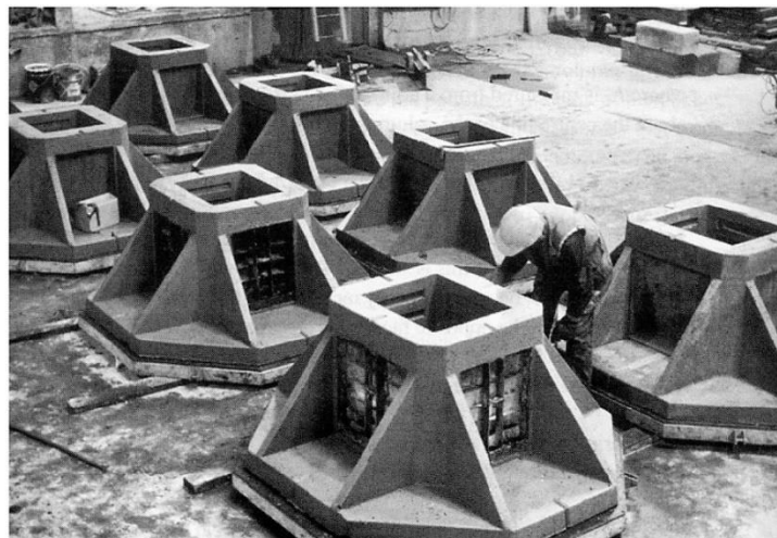
Figure 7.125 Precast concrete pocket foundation.
