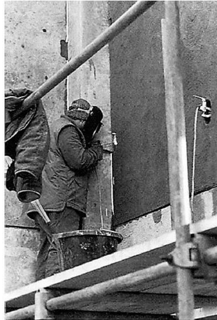
Shear jointing by site welding together steel plates in precast wall and column components.
