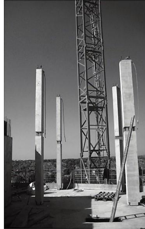
Precast columns with openings for in situ stitching to beam and/or slab connections. (Courtesy of HSP Consulting, Nottingham, UK.)
