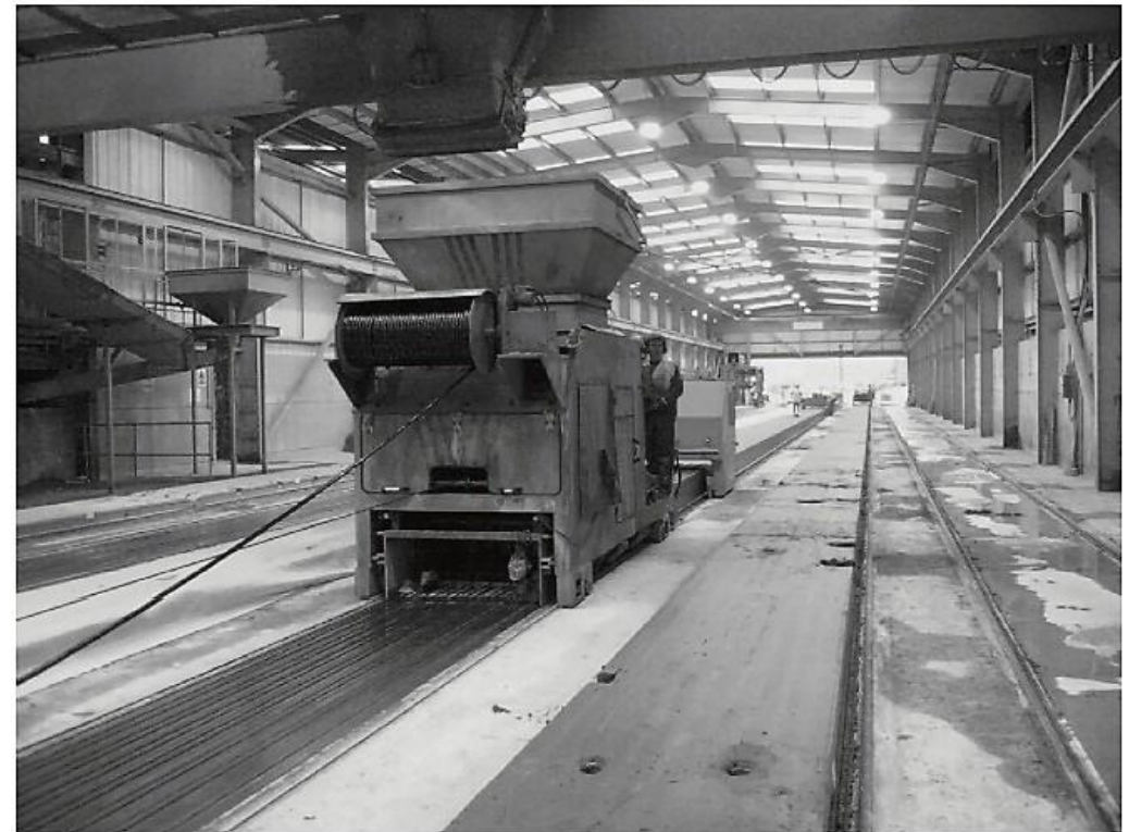
Long line slip form of prestressed hollow core floor slabs, at Bison Manufacturing, United Kingdom.
