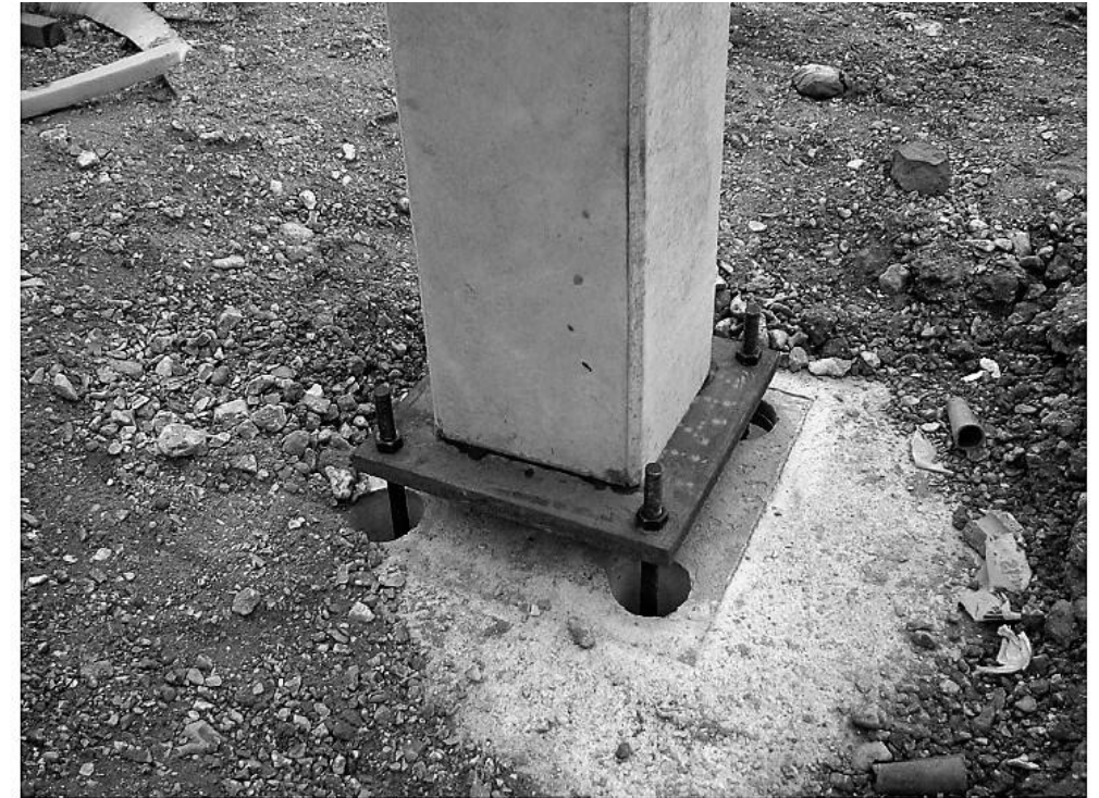
Figure 10.4 Column-to-foundation connection using extended steel base plate.
