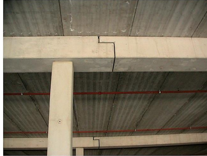
Figure 7.3 Reinforced concrete inverted-tee beams designed with a scarf joint at approximately 750 mm from the face of the column create a negative bending moment at the column that will reduce the depth of the beam.
