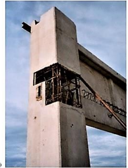
Figure 7.69 (a) Sliding plate connector steel plate is expressed from the beam after casting, and (b) is received into the steel box slots in the column.
