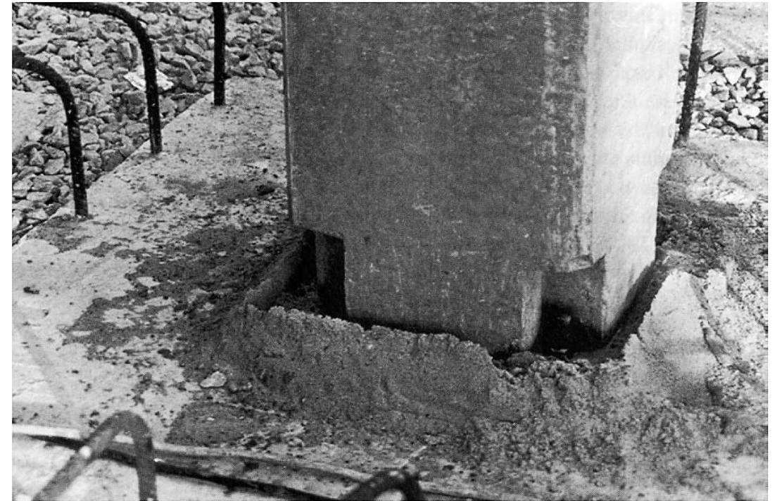
Figure 7.137 Column-to-foundation connection with flush base plate.
