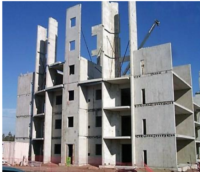
Forming the stability of multistorey frames using discrete structural elements. (Courtesy of Westkon, Melbourne, Australia.)
