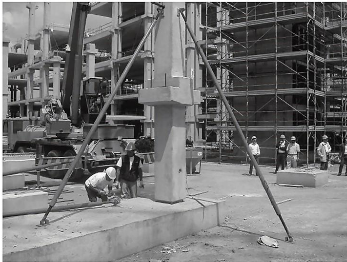
Stabilising columns with compression props.
