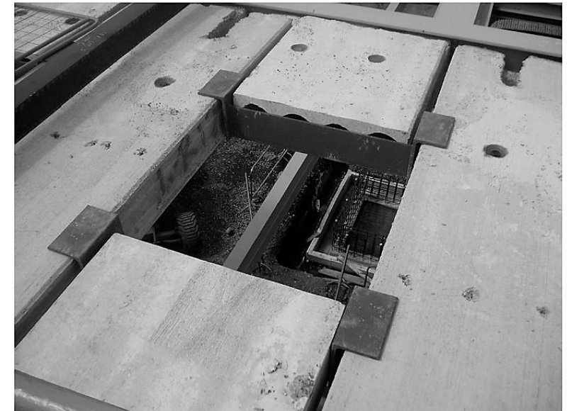
Steel trimmer angles are used to support units around large voids in hollow core slabs.
