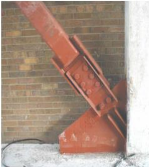
Friction damper in single diagonal bracing
