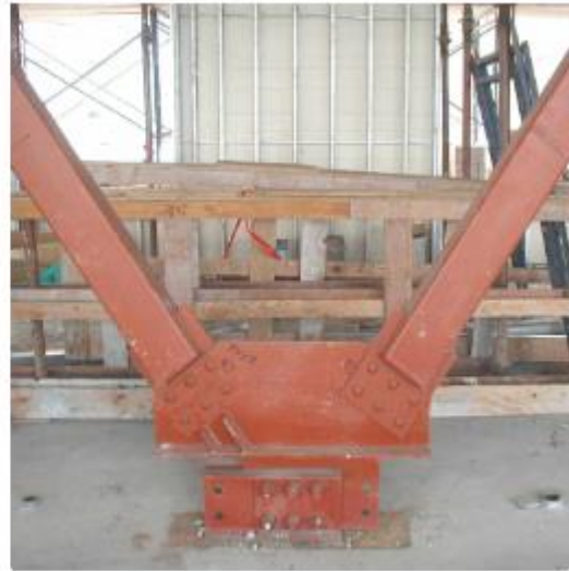
Friction damper in chevron bracing (inverted)
