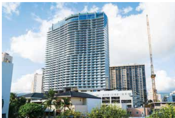
The Ritz-Carlton Residences Waikiki Beach, Phase 1, Honolulu, HI, was the PTI 2017 Project of the Year
