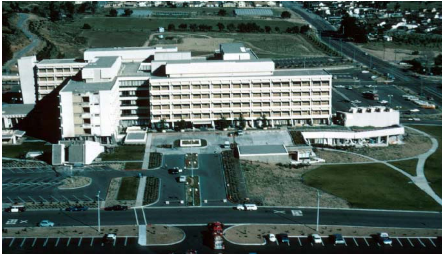
Two fallen and one tilted seismically-isolated (structurally separated) stair towers and the collapsed basement at Olive View Hospital.
