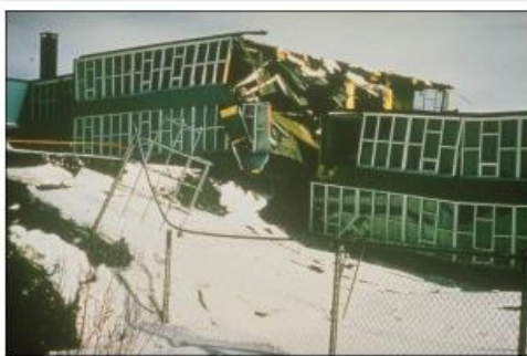
NORMAL FAULT, Government Hill School, March 27, 1964 Anchorage, Alaska
