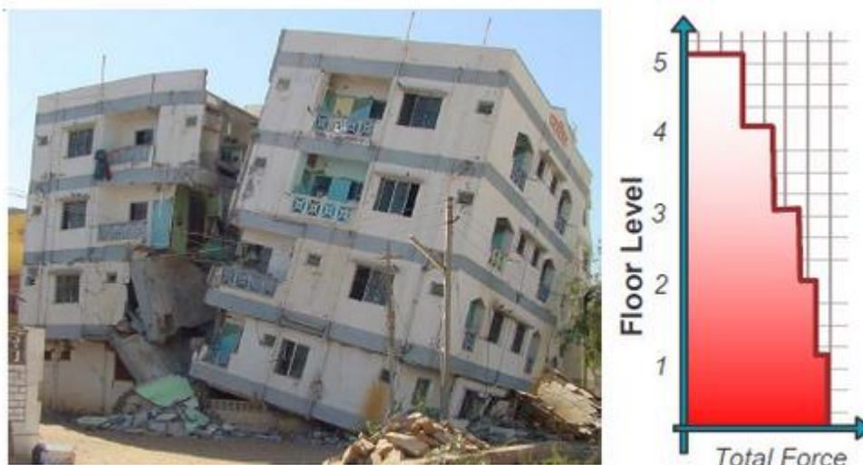
Figure 1: Total horizontal earthquake force in a building increases downwards along its height
