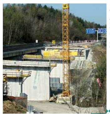
For the "Gschaid valley crossing" project at Altlengbach, outside Vienna, contractors Held & Francke turned to Doka for quality formwork equipment – in particular, Staxo load-bearing towers, which played a key role in the falsework construction. **Project data** Beam-and-slab bridge Gschaid, Austria
