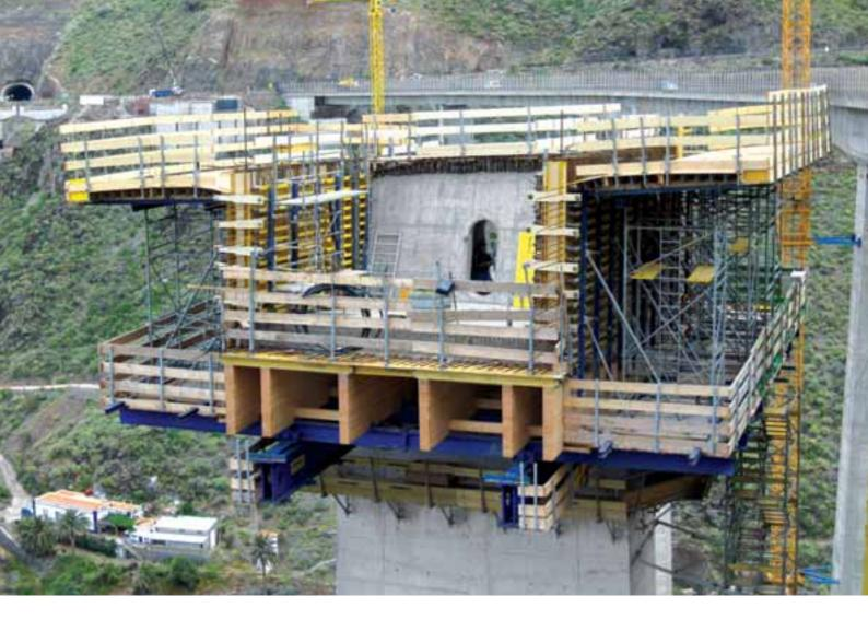
In close collaboration with the bridge planners, Torroja Engineria, and the client, UTE Guia-Pagador, a safe concept was elaborated for casting the pierheads, which are located 110 m above the ground. The Doka main support girder ensures safe working at all times. The main support girders are raised by crane and then pushed into place through the pier hydraulically. The various different inclinations and structure
