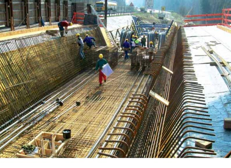
deck slab was cast using specially made Top 50 cover-slab elements supported on roller brackets. After the formwork had been struck, these elements were towed over the roller bearings of the roller brackets into the next casting section, as a single unit.
