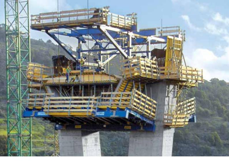
the tendons). Note that the V-shaped piers already had to be finished up to the level of the top of the deck slab, in order to be able to carry the cantilevering superstructure. This exact casting sequence is only possible thanks to proper planning and continuous liaison with the contractors.
