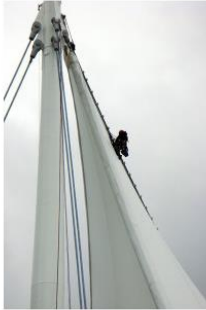
Figure 5. Inspection of ridge cable.
