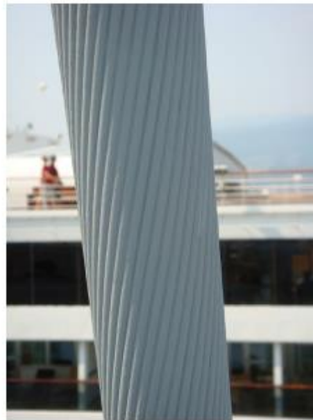
Figure 6. Applied coating after 6 years.
