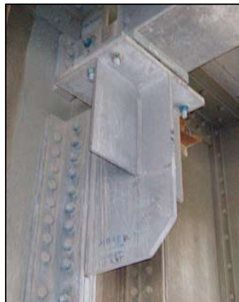
Figure 1: Installed seat bracket at Main Span.
