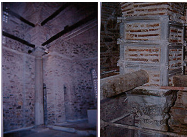
Fig. 4 St Panteleimon Church, Thessaloniki. Metallic braces for confinements of small part of pier above the column capital (Photograph courtesy of Prof. Ch. Ignatakis and Prof. K. Stylianidis)
