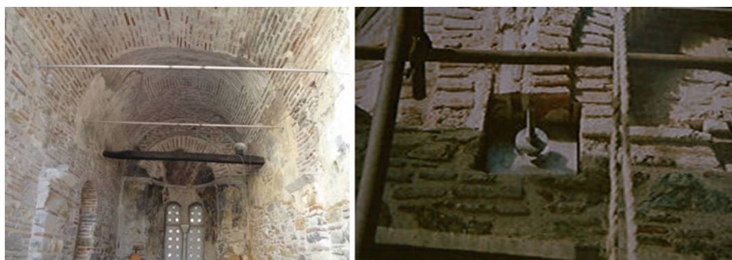
Fig. 3 St Panteleimon Church, Thessaloniki. Substitution of wooden tierods with stainless steel ones (Photograph courtesy of Prof. Ch. Ignatakis and Prof. K. Stylianidis)
