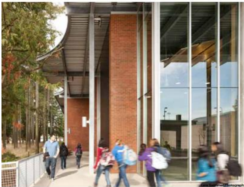
A Galvanized steel-framed cantilevered canopies highlight the new addition.
