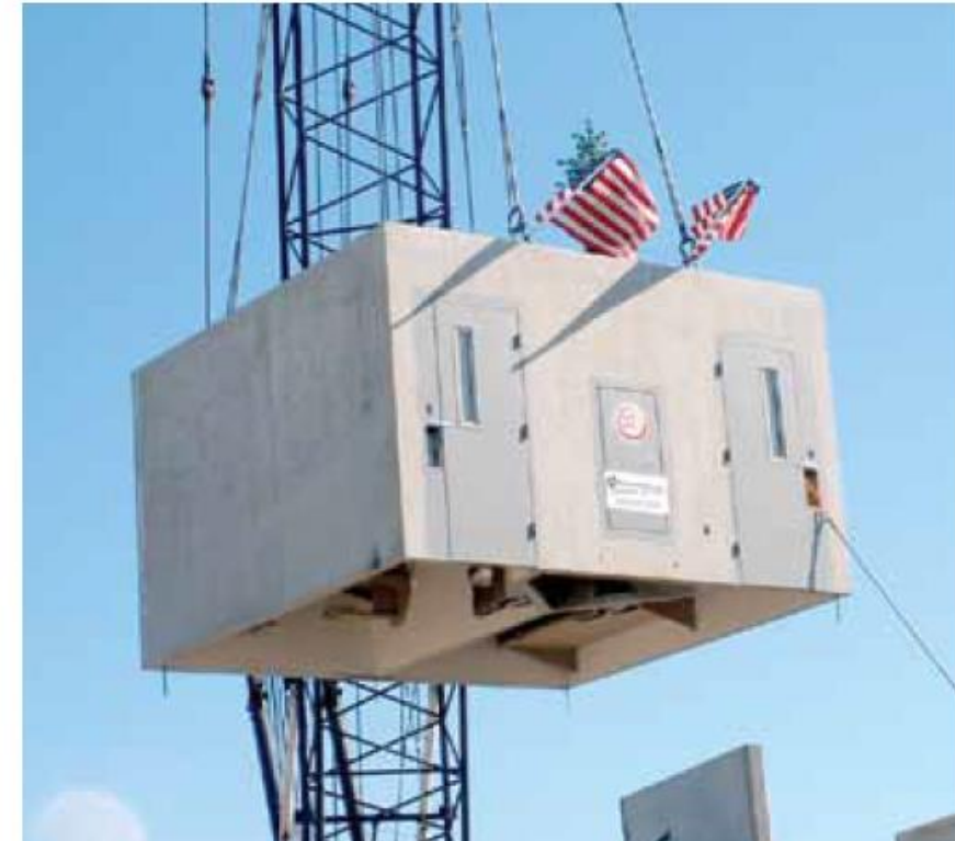
Fig. 1.2.16 A precast concrete double-cell module is lifted into place, complete with furnishings installed.
