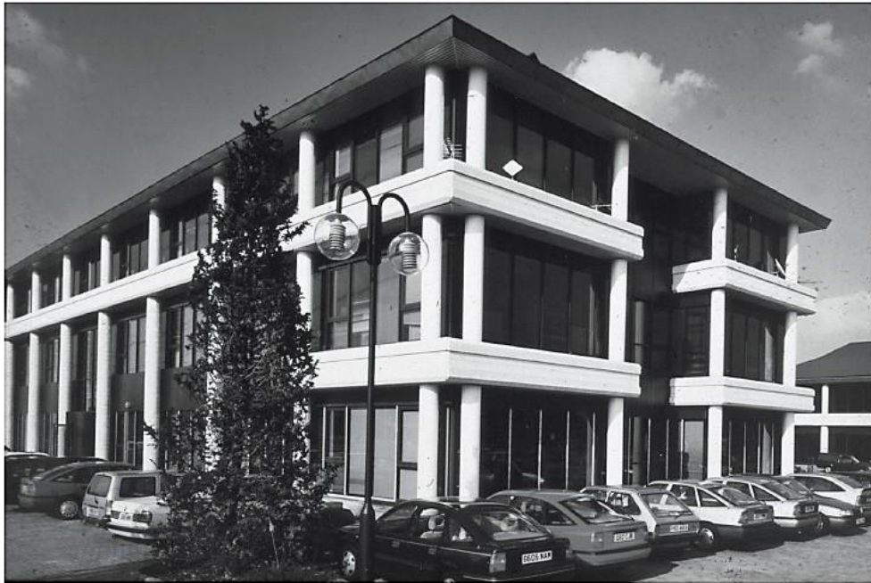
Precast 'skeletal' structure with integrated architectural columns and spandrel beams, Reading Business Park. (Courtesy of Trent Concrete Ltd., UK.)
