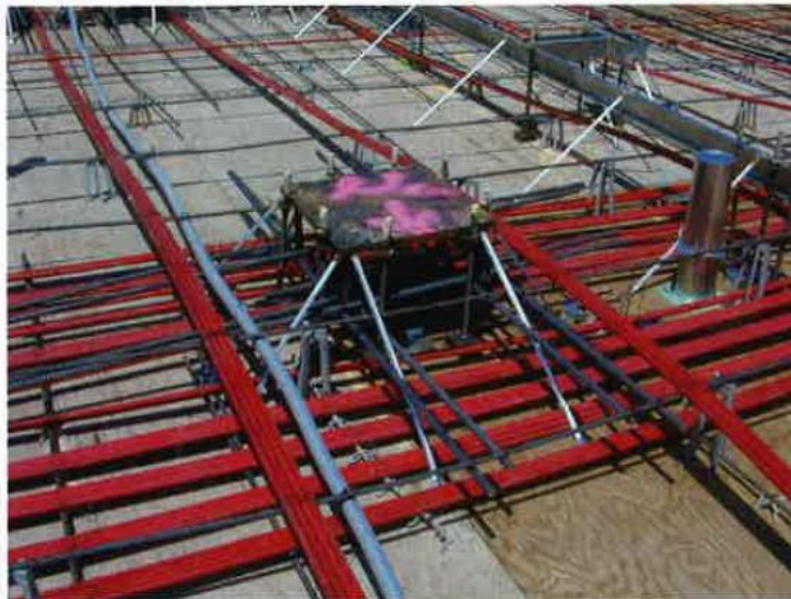
(a) Base plate of steel columns planted on PT slab (P136a)
