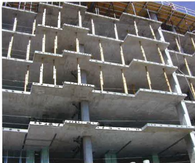
FIGURE 2.2E-1 Beamless Flat Slab Construction Using Post-Tensioning (P134)
