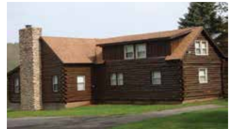
Figure 7. Log cabin after wall repair.
