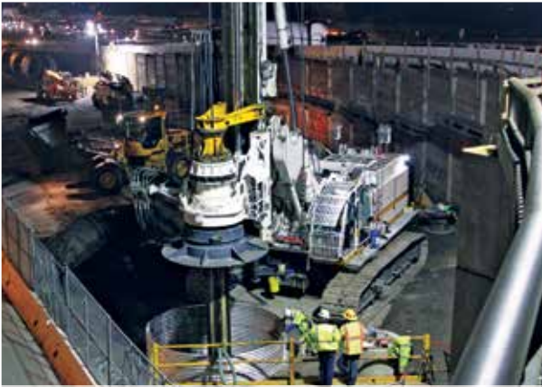
Drilled shafts provided deep foundations for bridges along a freeway.
