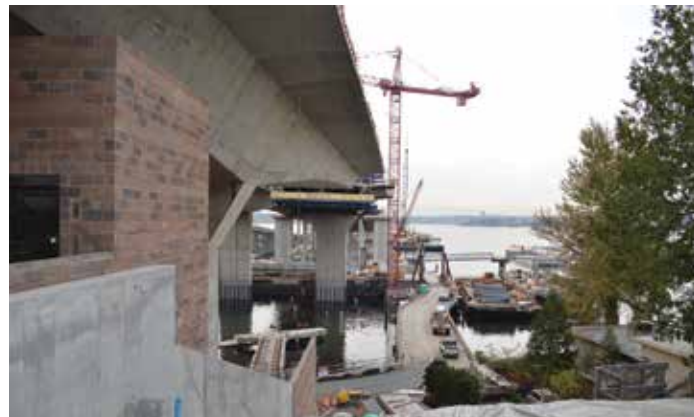
Land to water access trestle.
