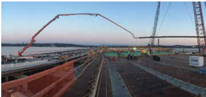
Placing concrete from the mainline to BCD raft. Courtesy of KGM.
