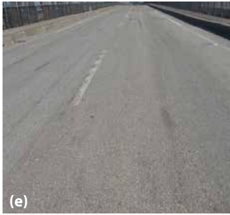
Figure 4. Service state of five retrofitting schemes on the Mafang Bridge after nearly 4 years of service (photos taken in Sep. 2015). (a) Stone asphalt concrete; (b) Epoxy asphalt; (c) Sandwich plate system; (d) Polymer modified asphalt concrete; (e) Proposed LWCD.
