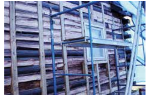
Figure 6. Staging of repair in progress.
