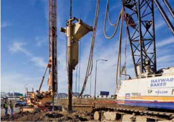
Vibro replacement for ground improvement beneath bridge retaining walls.
