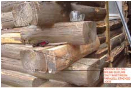
Figure 4. Log profile; note reveal for the spline.
