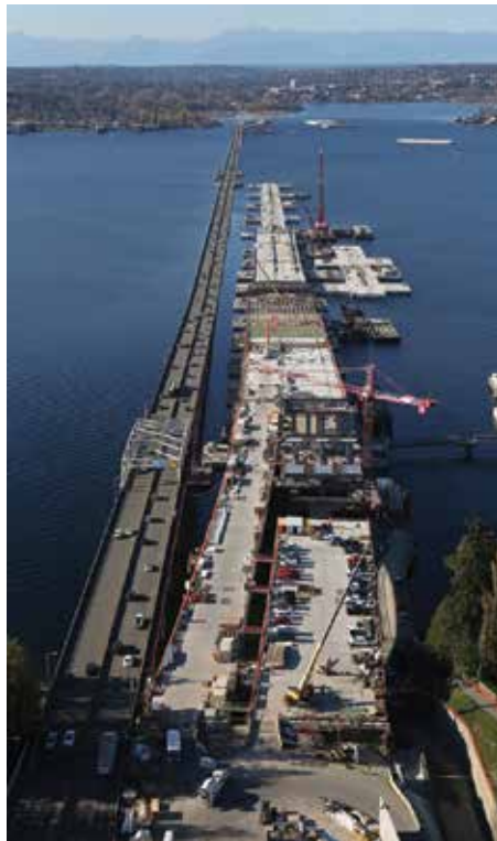
Aerial view of mainline bridge and BCD raft pontoon.
