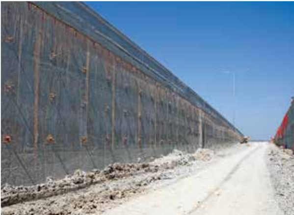
Soils nails to support an elevated freeway.
