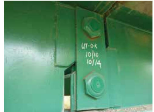
Figure 1. Pin-and-hanger assembly.
