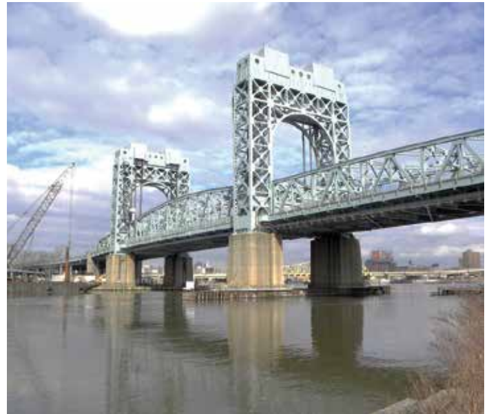
Figure 3. Harlem River Lift Bridge. Courtesy of T.Y. Lin International.
