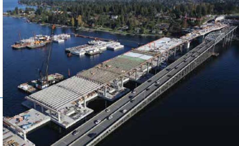
Aerial view of State Route (SR) 520 Evergreen Point Floating Bridge high-rise superstructure under construction.
