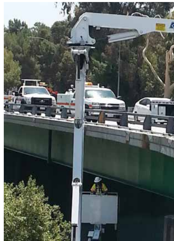
Figure 2. Under bridge inspection truck (UBIT).
