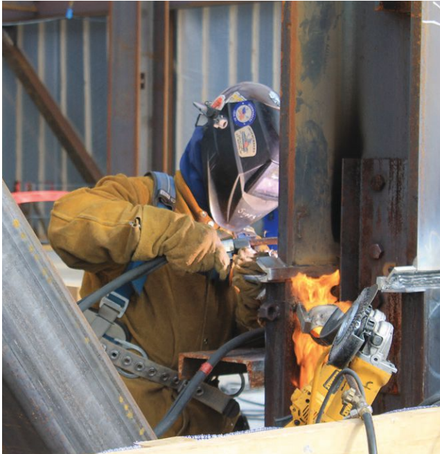
▲ Personal protective equipment is the last line of defense when it comes to safety.
