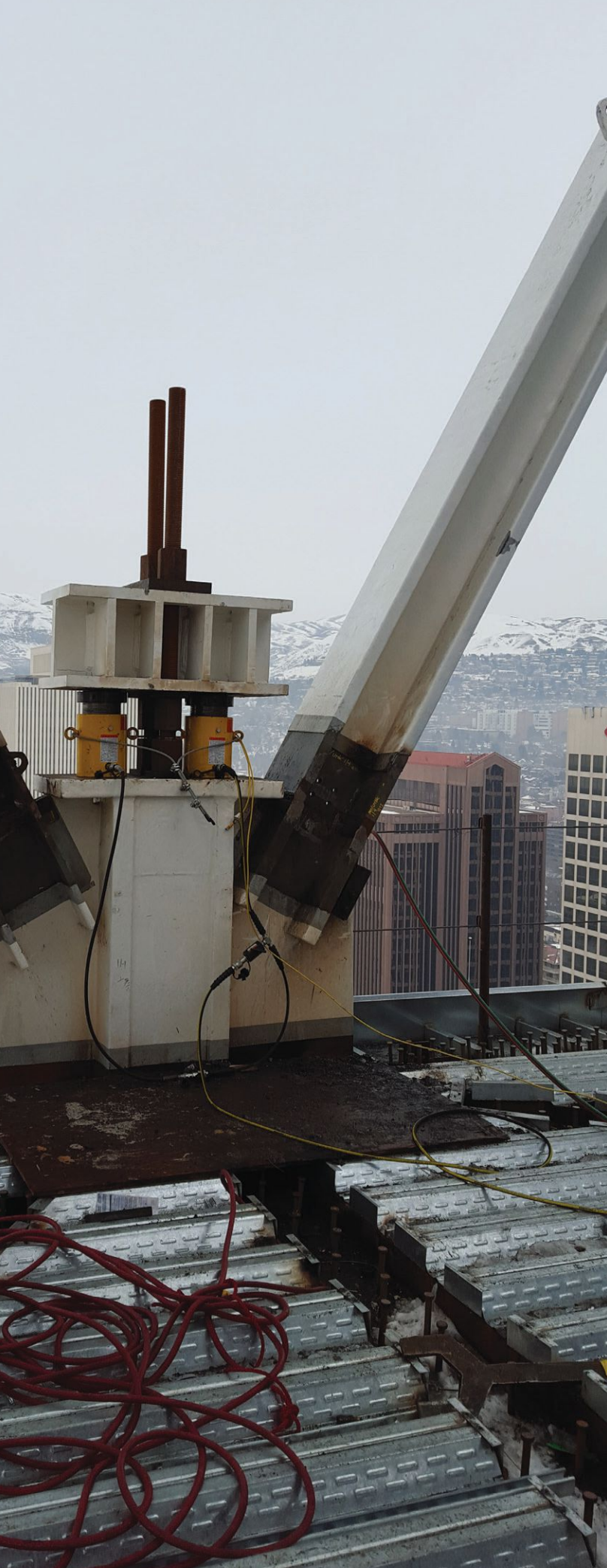
◀ Jacking adjustments at the roof node.
