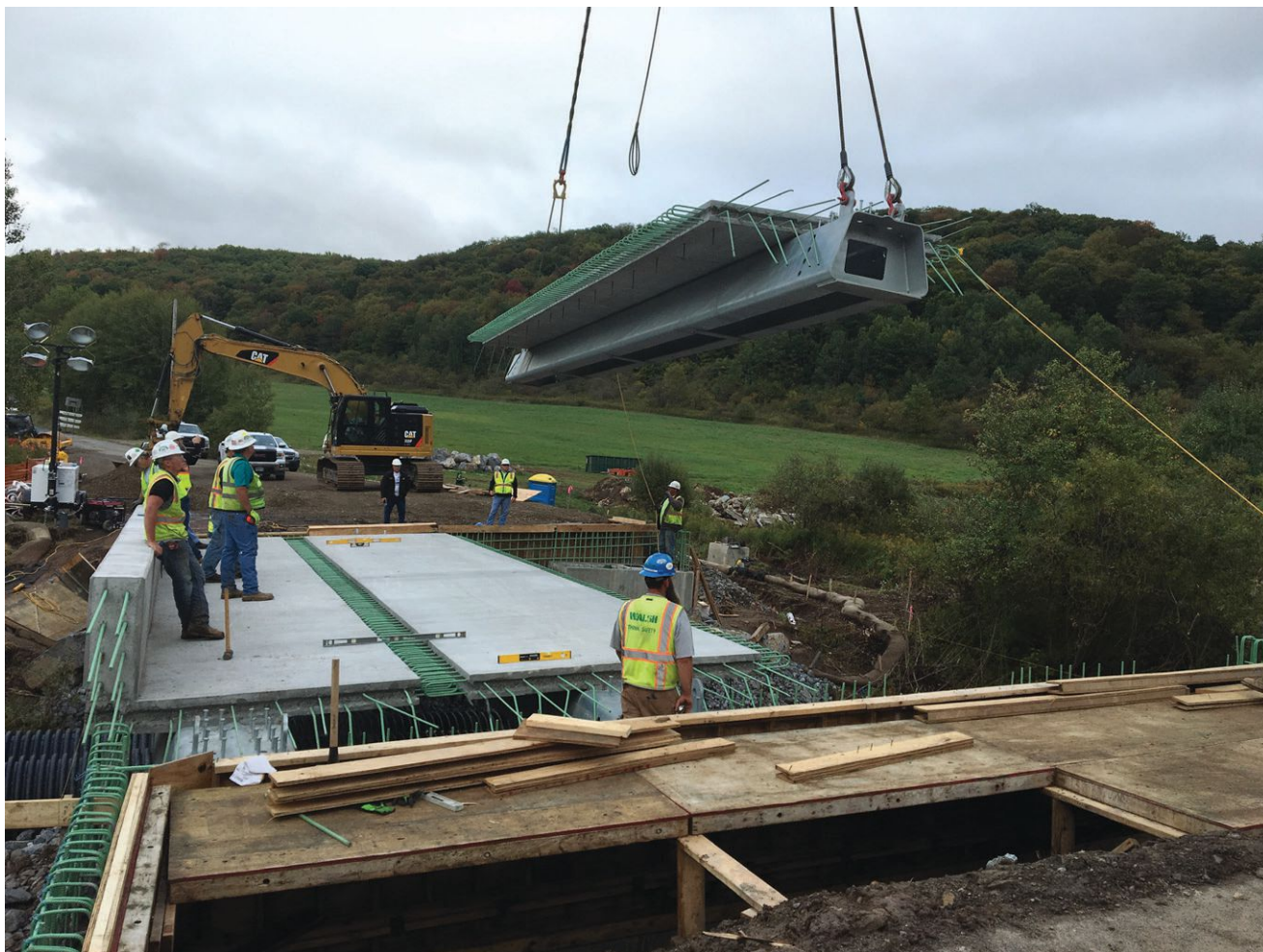
▲ Installing the third section.
