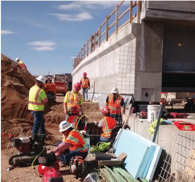
▲ Wing wall construction, following the slide.
