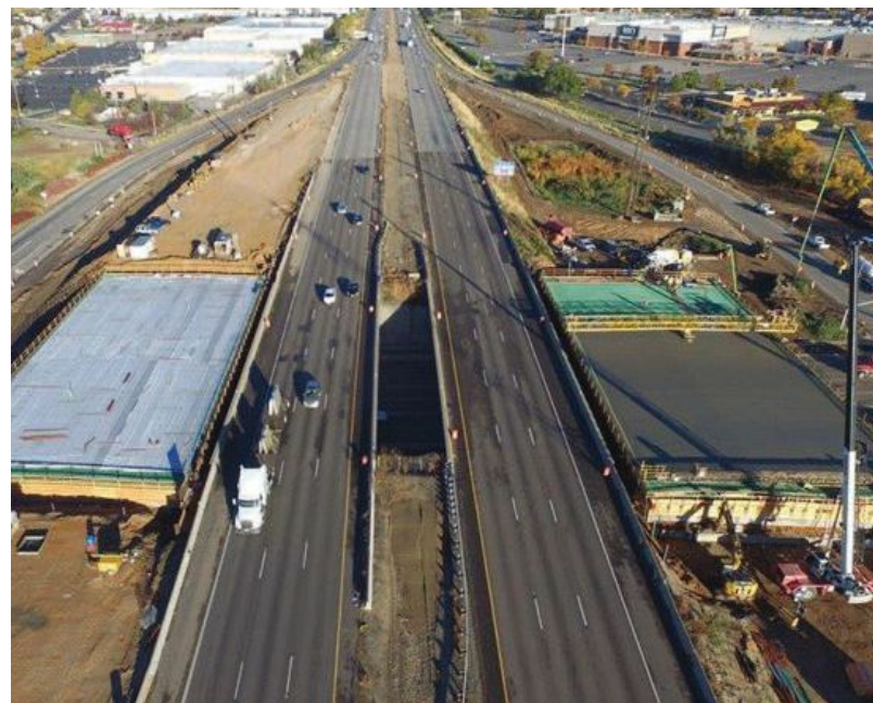
▼ The new superstructures were built next to the existing ones.
