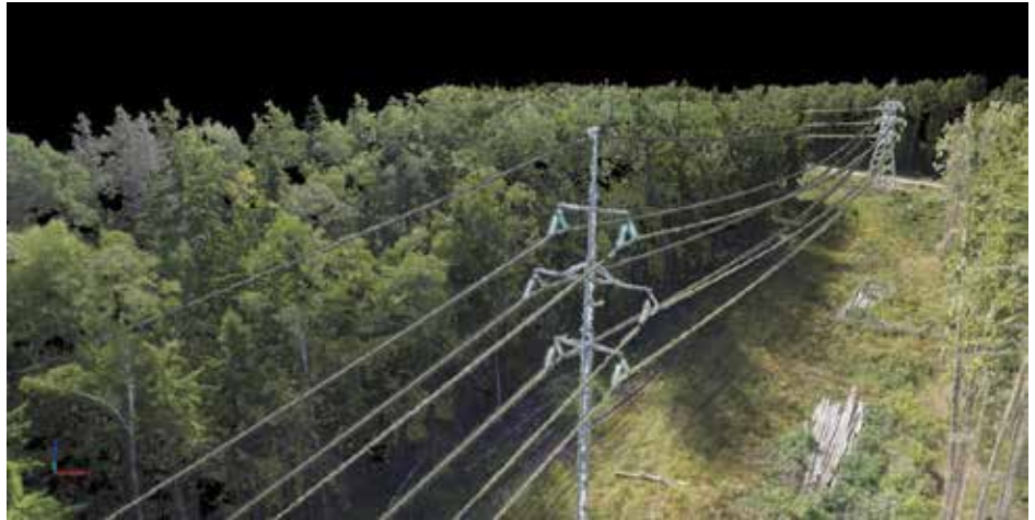
Figure 1. Aerial scan of transmission line using photogrammetry.
