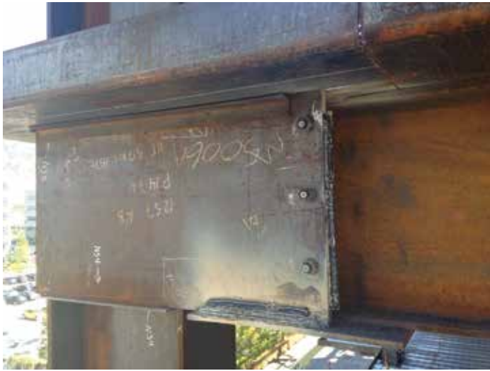
Figure 2. SidePlate connection.
