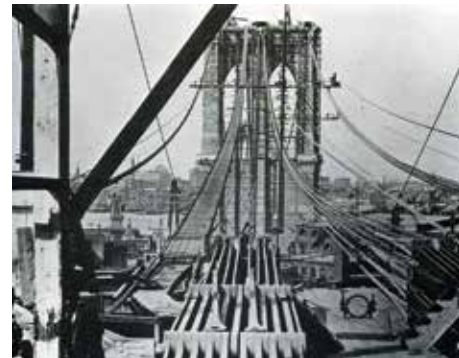
Cable spinning, showing anchor chains, foot walk, adjusting cross walkways, and tower.
