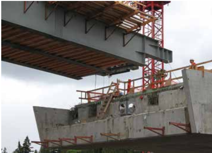
Figure 4. Girders being erected over the trailer hitch.
