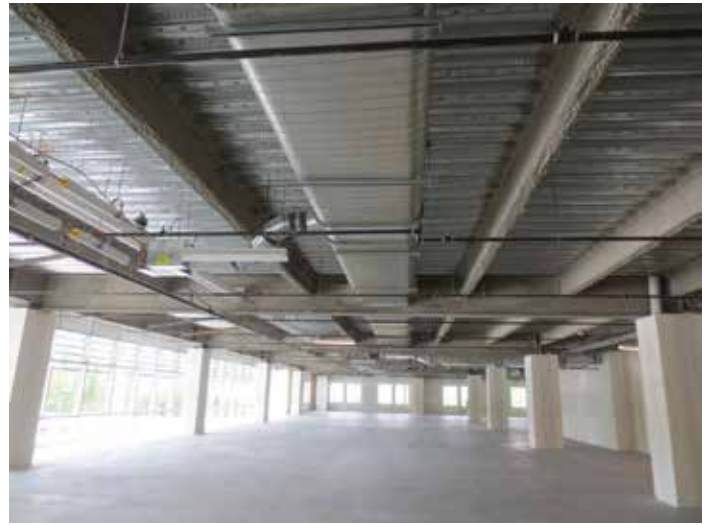
Figure 3. Steel girder web openings.
