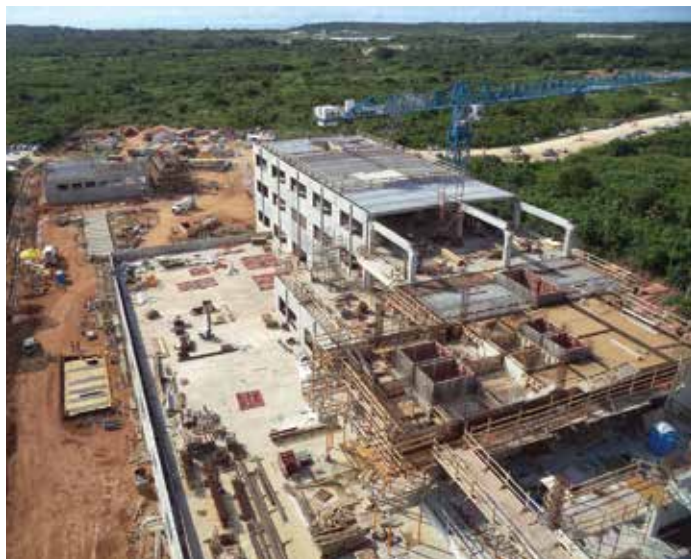
View from tower crane during construction. Courtesy of dck pacific guam, LLC.
