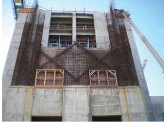
Diagonal reinforcement at the special shear wall.
