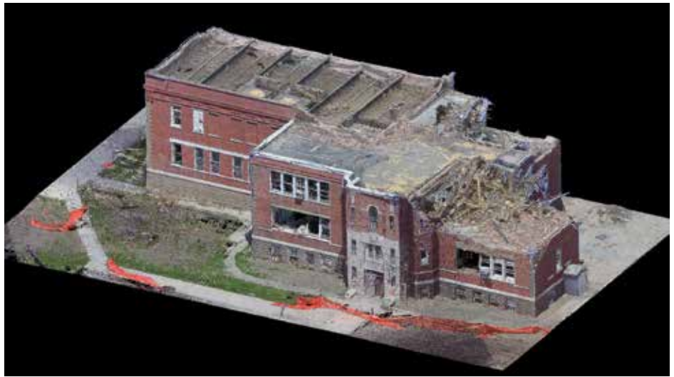
Figure 2. LiDAR scan of damaged school following a tornado. Courtesy of Richard Wood from the University of Nebraska-Lincoln.
