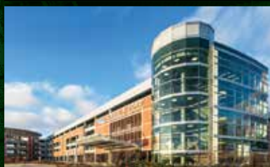
FORD INT. AIRPORT PARKING DECK / GRAND RAPIDS, MI
