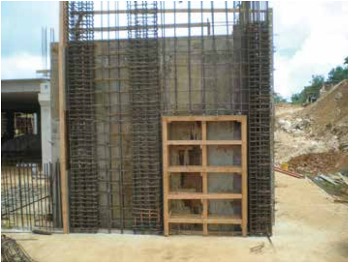
Boundary element reinforcement at the special shear wall.
