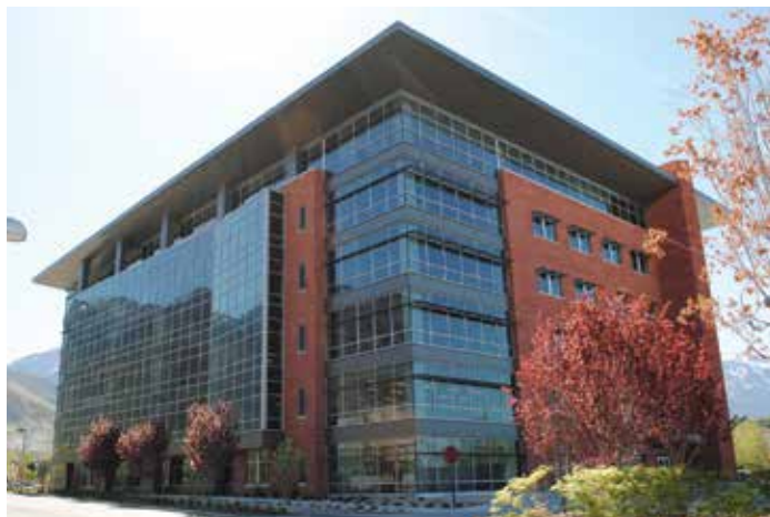
Figure 6. Cut sandstone façade and full height windows.
