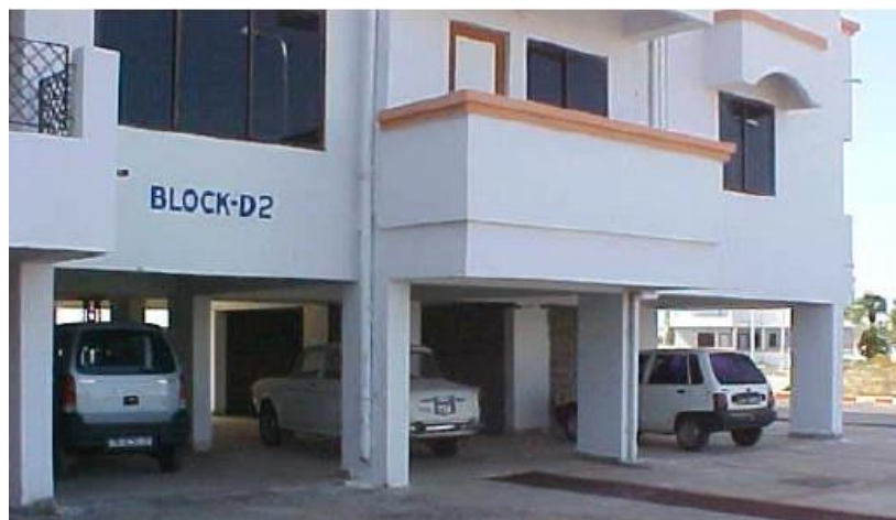
Figure 1: Ground storeys of reinforced concrete buildings are left open sometimes to facilitate parking.
