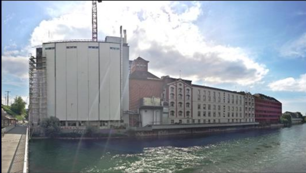
Existing silo: 38 meter high 50 years old
