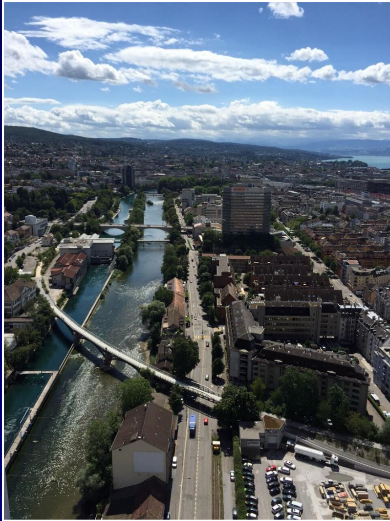
Photo from top of silo: River with train viadukt
