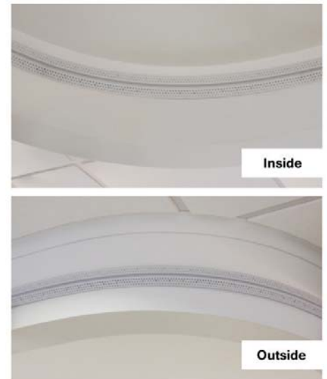
The flexibility of vinyl reveals also allows them to conform to curved walls and soffits. The minimum inside and outside radius is determined by the width and depth of the reveal, the 1/4" x 1/4" reveal being the most flexible.
