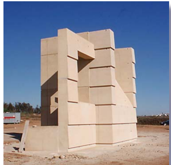
Figure 2: Cathedral of Our Lady of the Angels, Los Angeles, CA, Mock-up of different formed elements, including angled wall. Contractor Morley Builders
