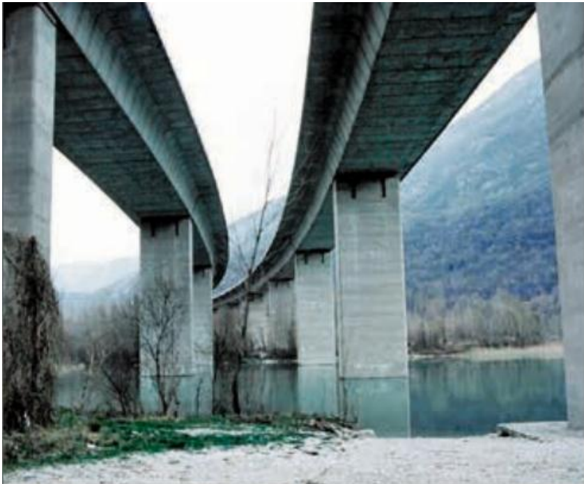
• ITALY -- Somplago Viaduct, 1974 buffers, Europe's first seismically isolated bridge, 1974
