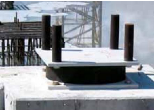
EIs as installed in the "Da Luz" Hospital, Lisbon, Portugal.
