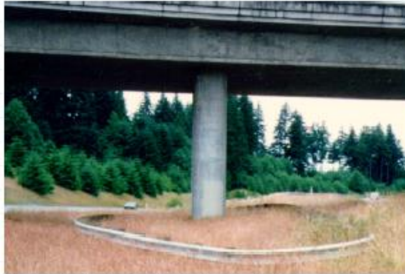
Guardrail around a bridge pier
