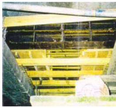
Placement of temporary reaction devices between girders.
