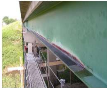
(f) CFRP plate installed.
