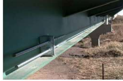
CFRP Rods on span
