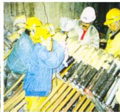
Injection of mortar into the tendon mounted anchorages.
