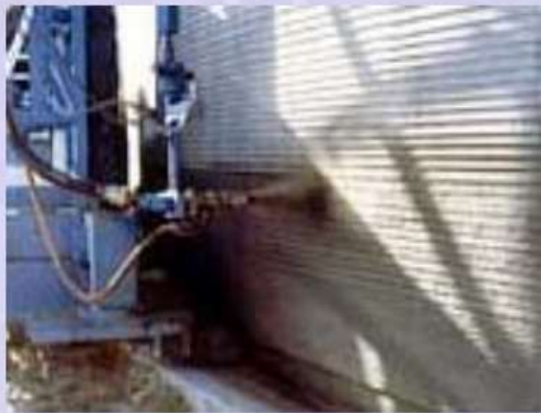
(c) Shotcrete operation
