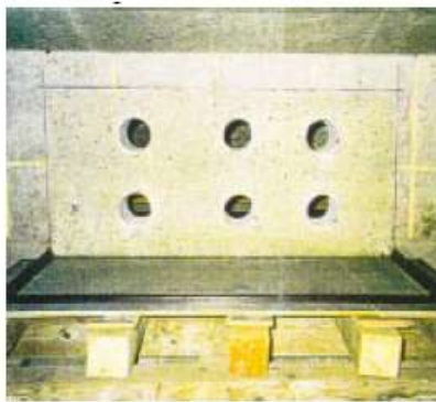
Drilling of holes into girders for the introduction of aramid tendons.
