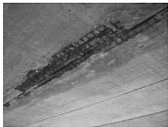
Cracks in slab.
