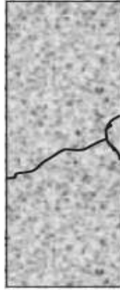
Cracks due to eccentricity
