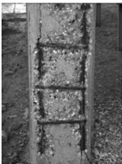
Pier reinforcement corrosion
