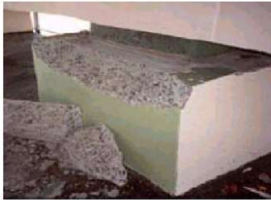
Damaged concrete pedestals of the elastomeric bearing of the New Surajbadi Highway Bridge.
