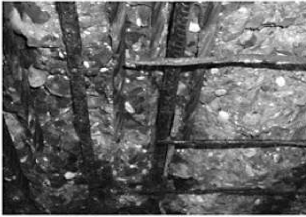
Broken reinforcement in girder.
