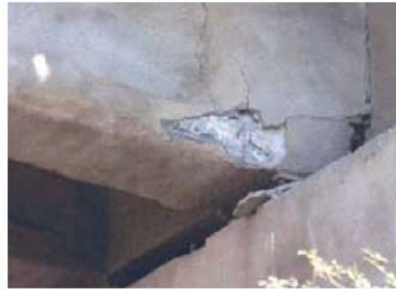
Damaged soffit of the girder at the span ends of the New Surajbadi Highway Bridge.
