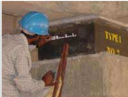
Lead Rubber Bearing (LRB)
