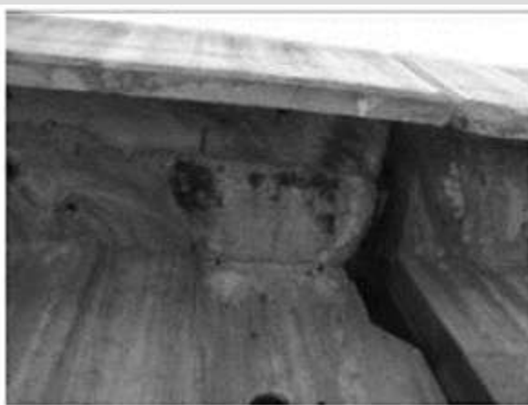
Leakage through Expansion joint.
