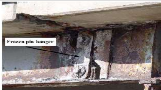
a) Corroded Expansion Joint Details
