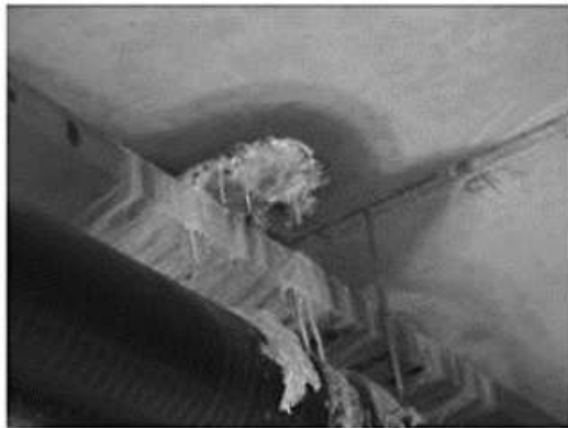
Efflorescence from freezing-and- thawing deterioration.
