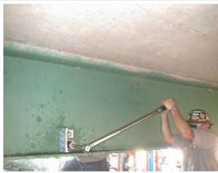
(a) Installation of anchorage assembly
