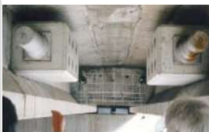
End view of anchor blocks with external cables and anchorages.
