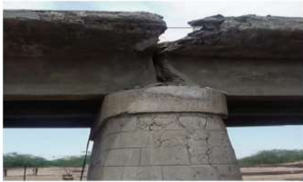
Failure of the girder end and expansion joint of a bridge between the towns of Gandhidham and Bhachau.
