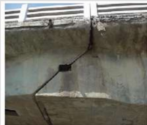
Failure of in-span hinge and traffic railings at Old Surajbadi Highway Bridge.
