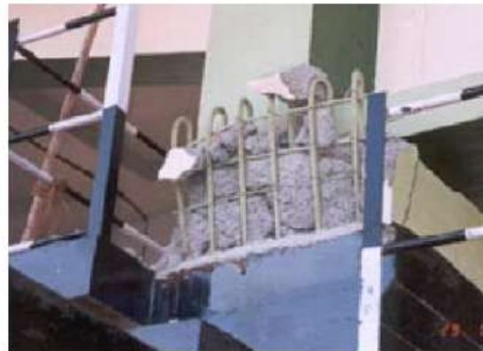
Damaged reinforced concrete stoppers showing poor bond between the epoxy-coated rebar and the adjoining concrete at the New Surajbadi Highway Bridge.
