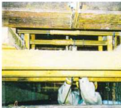
Cutting of tendons between girders after cure of concrete in anchor blocks.
