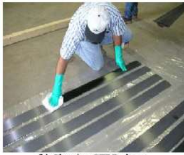
(b) Cleaning CFRP plates
