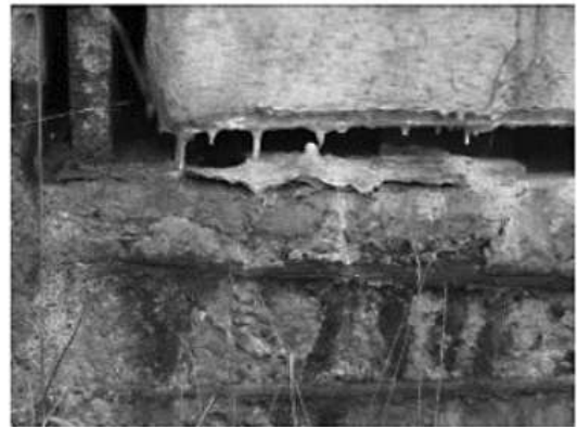
Reinforcement corrosion on abutment wall.
