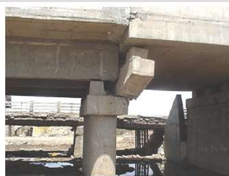
Failure of crossbeam of a bridge at the village Vondh.
