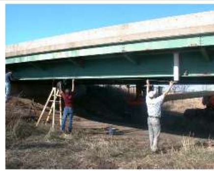
(b) Placement of CFRP rod
