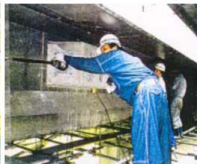
Installation and jacking of external steel cables.
