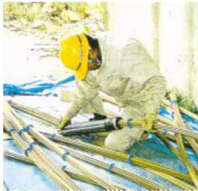
Preparing the anchorage (bond-type)
