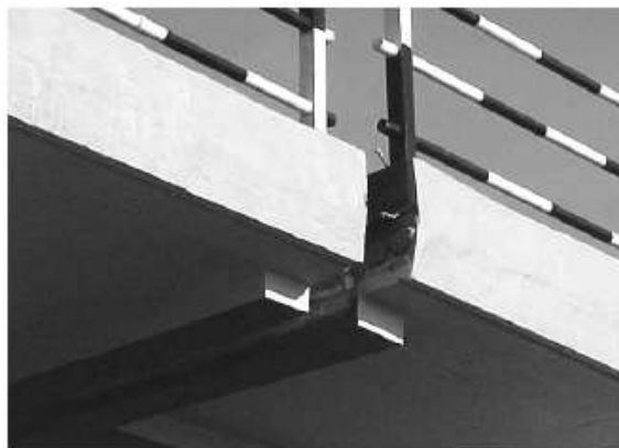
Transverse displacement of the superstructure decks of the New Surajbadi Highway Bridge.
