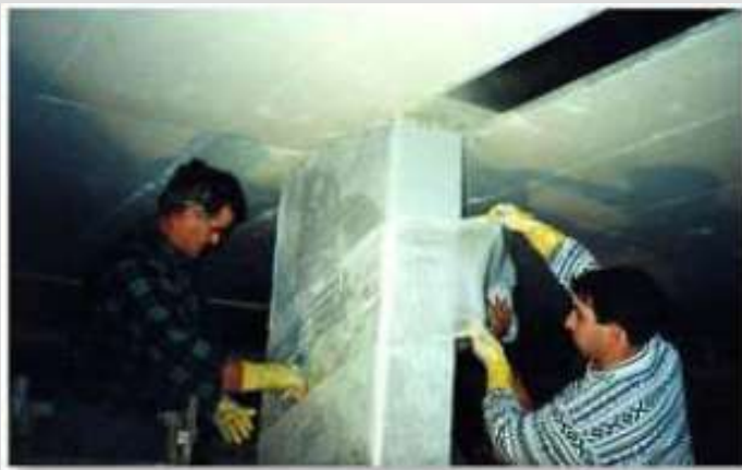
Installation of CFRP Plates on Bridge
