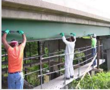
(e) Placement of CFRP plate
