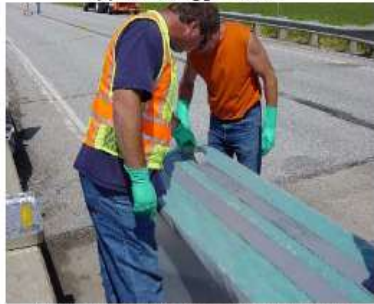
(c) Epoxy application on CFRP plates
