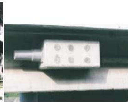
View of anchorage block showing position of 6 AFRP tendons.
