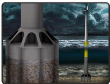
Fig.-1 Skirt Suction Foundation
