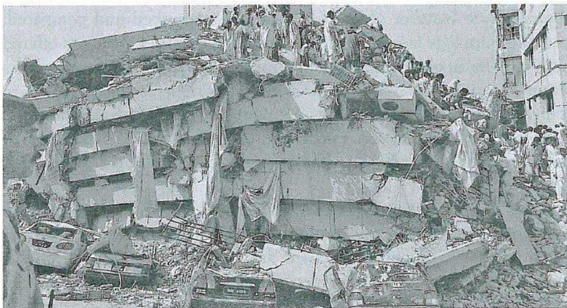
Fig. 2.1 Pancake-type collapse of a ten-storey building triggered by an earthquake (Islamabad, 2005)
