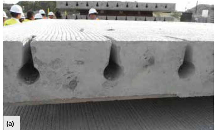
Fig. 5: Barra Glide® dowel system, showing the partially open narrow slots at the surface of the precast panel. Here, the worker is using a small diameter bar to push a dowel into the adjacent panel
