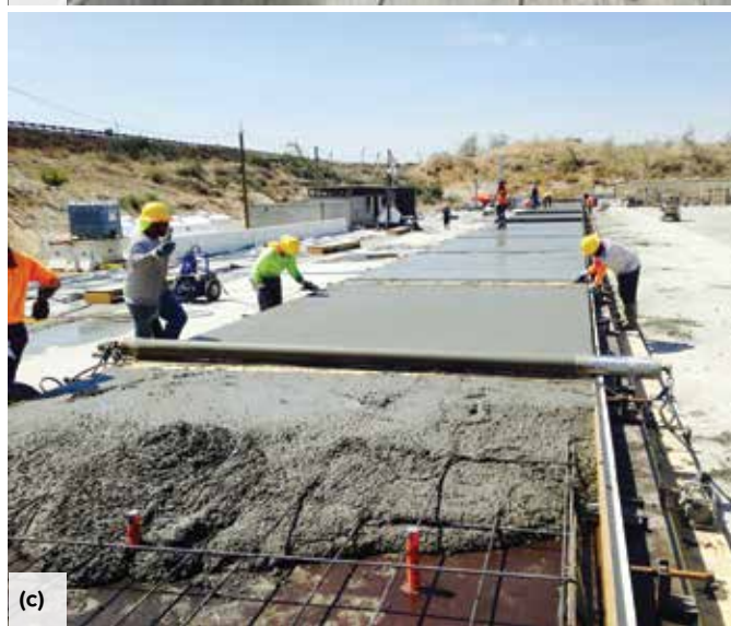
Fig. 8: Panel production using outdoor prestressing beds: (a) view of a prestressing bed; (b) panel hardware including prestressing tendons; and (c) concrete placement
